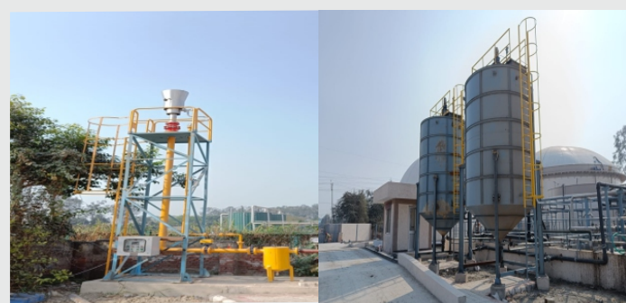
Biogas Burner & Sedimentation Tank
